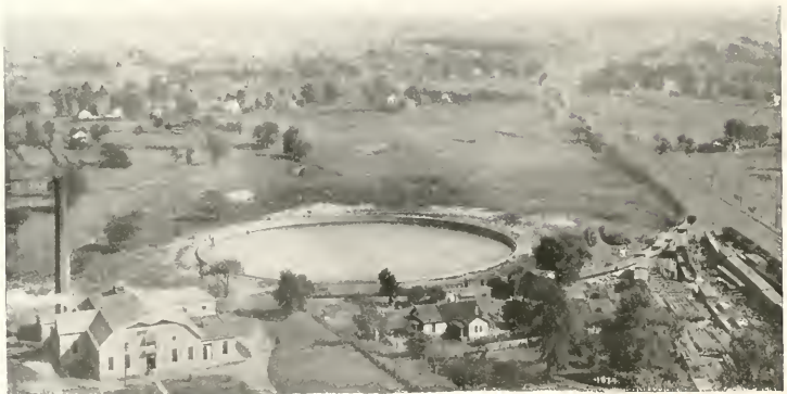
Reservoir Bloomington's Municipal Water Plant
