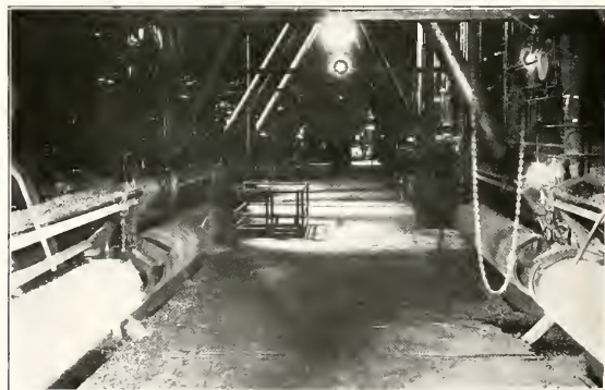
Boiler Room of the Bloomington and Normal Railway and Light Company
