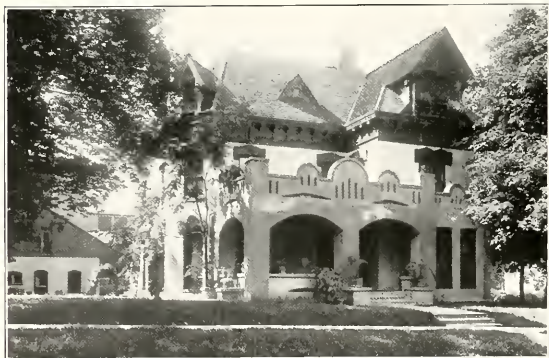
Residence of C. L. Hills, 406 W. Jefferson Street
