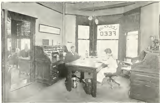
Sales Manager's Office and Portion of President's Office
