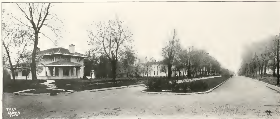
BROADWAY BOULEVARD EXTENDING NORTH OF CEDAR CREST
