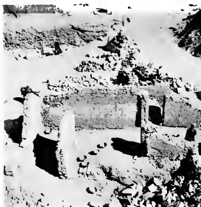
Brick House in southern Court.
