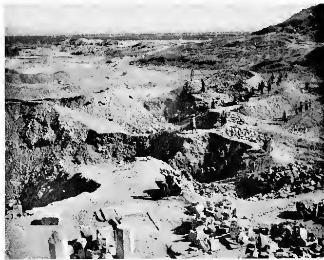
Digging the Great Trench, Nov. 1904.
