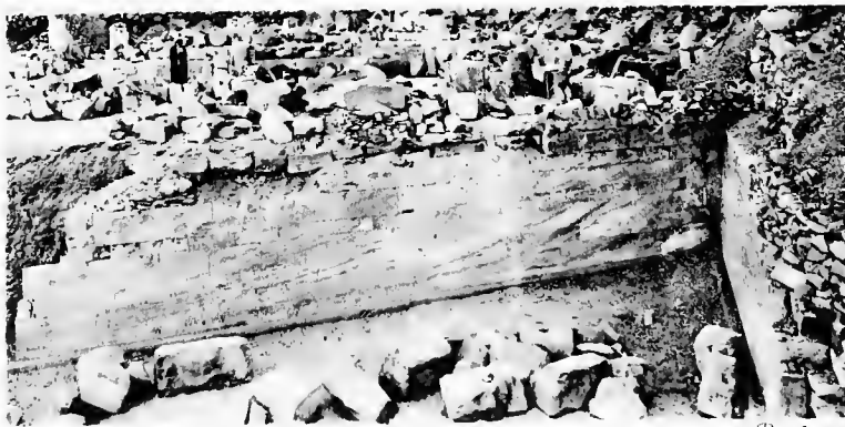
North lower cocert showing sharp angle of walls. Borchardt
