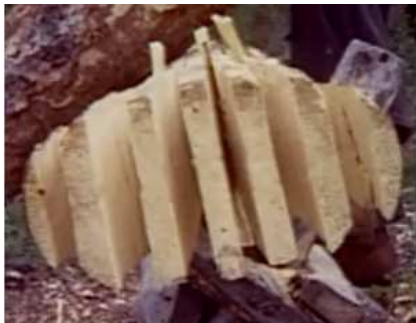
Here Proenneke is splitting the log into planks, making the hinges, and hanging the outhouse door.
