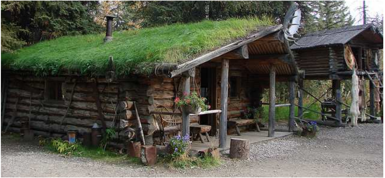
Here is a typical small cabin, with elevated food cache. Note the roof poles, visible under the extended porch.
