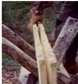
Here Proenneke is splitting the log into planks, making the hinges, and hanging the outhouse door.
