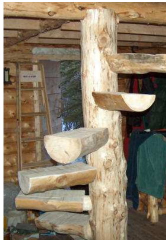
If the traditional log ladder doesn't appeal to you, check out this interesting spiral log staircase.
