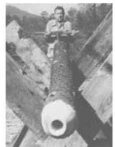
Running Water: Water can be supplied to your cabin from an uphill source, by using log gutters, or log pipes.
