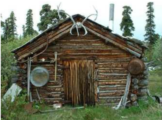
The number, size, and location of cabin doors and windows can be arranged in any manner that you like. Some trapping cabins have been made with no windows, and tiny doors, to keep bears from breaking in.
