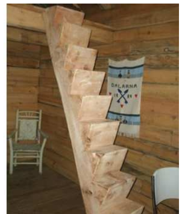
Ladders: Logs have been notched to create log ladders for hundreds of years. Plank steps are an optional upgrade.
