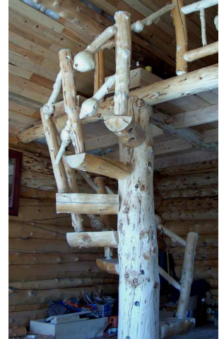
If the traditional log ladder doesn't appeal to you, check out this interesting spiral log staircase.
