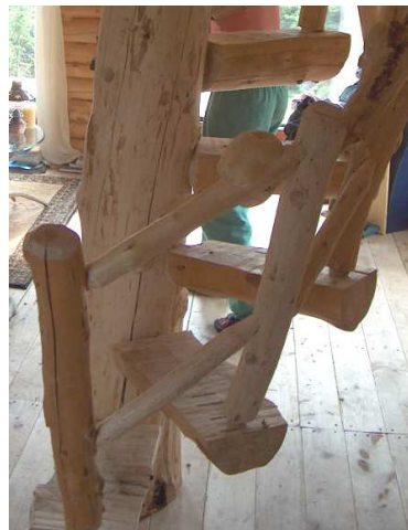
If the traditional log ladder doesn't appeal to you, check out this interesting spiral log staircase.
