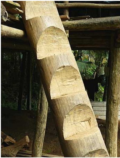
Ladders: Logs have been notched to create log ladders for hundreds of years. Plank steps are an optional upgrade.
