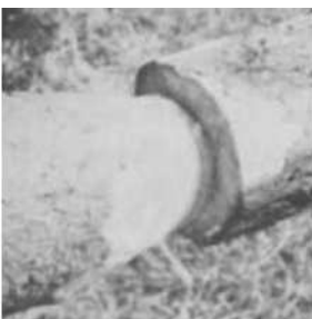
Log pipes are made by drilling out the center of logs with a long auger, and tapering one end, to fit in the next log.
