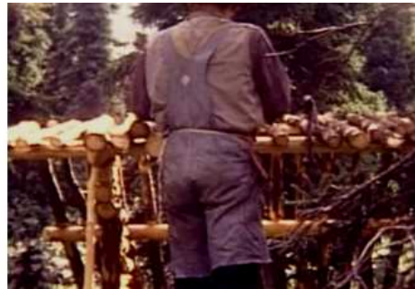
Once he had furniture, he gathered more materials and made an outhouse out of poles. He also split up a log to make the planks for the outhouse door, and made hinges from flattened tin cans, using nails for the hinge pins.
