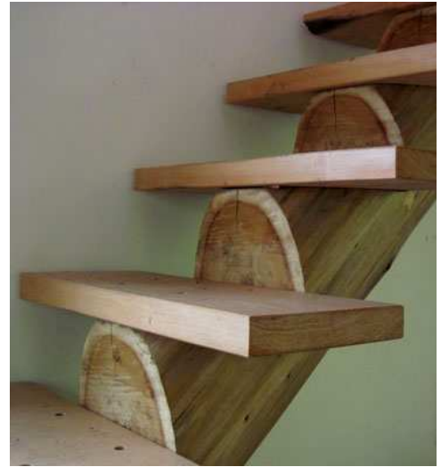
Ladders: Logs have been notched to create log ladders for hundreds of years. Plank steps are an optional upgrade.
