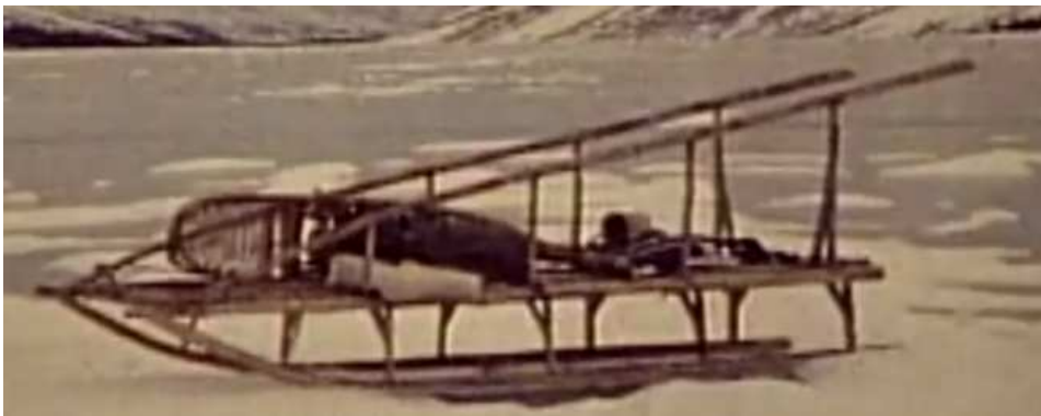
Here is the finished sled, which can be pushed from behind, or towed with a rope, or a team of dogs.
