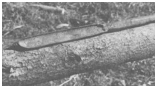
Running Water: Water can be supplied to your cabin from an uphill source, by using log gutters, or log pipes.
