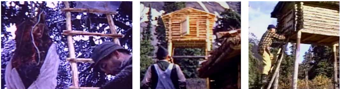
Proenneke stored his smoked meats by hanging them up in a tree, wrapped in cloth, until he had time to build an elevated food cache. The cache was a tiny cabin on stilts, used to keep food safe from bears and other animals.
