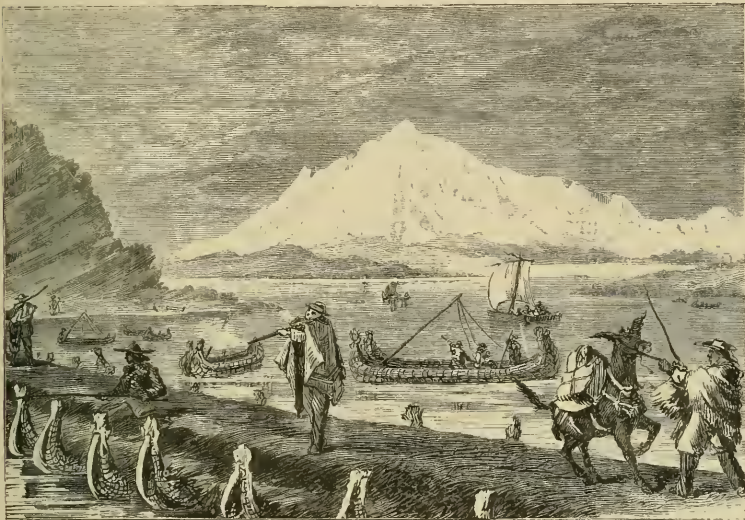
TOTORA BRIDGE OVER THE OUTLET OF LAKE TITICACA.
