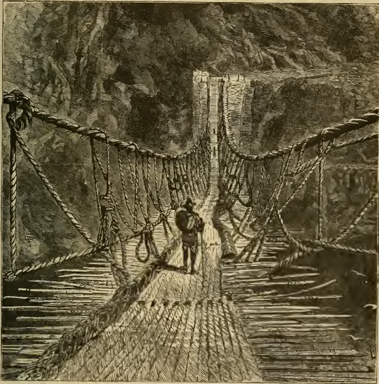
LOOKING ACROSS THE BRIDGE.
